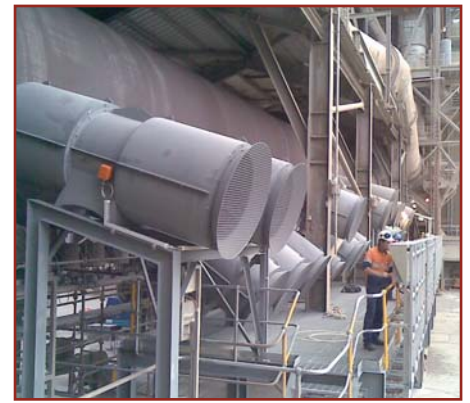
Air cooling system with in/out sound attenuation
